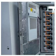
Frequency inverter, 60Hz to 50Hz
